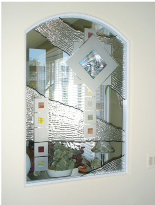
Slumped Glass Interior window with fused ink inlay. Custom Art by In house artist Larry Cripps
